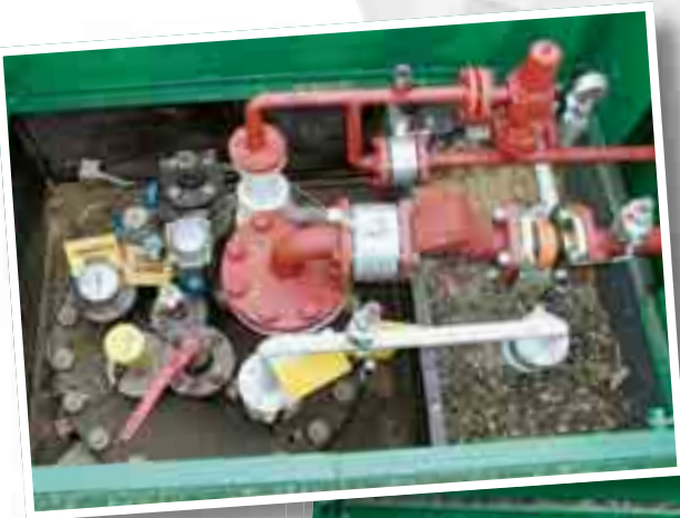
Underground autogas installation with one tank. Corken's autogas series pump replaced a previously installed submersible design.
